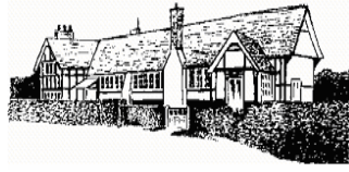
Husborne Crawley Lower School
